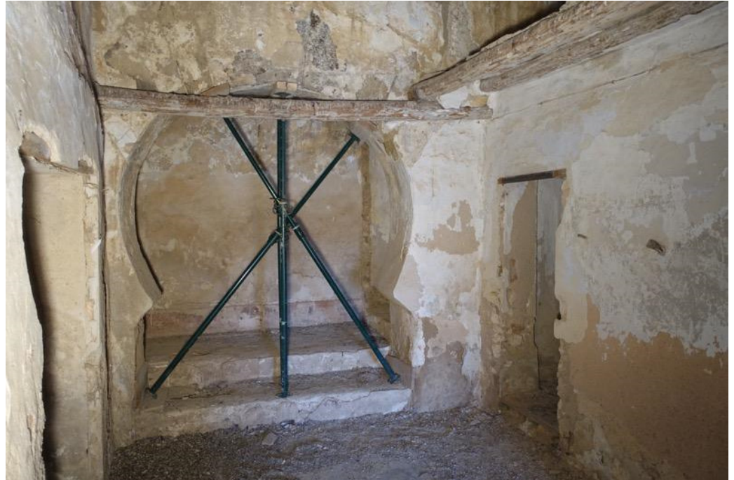
Figure 13. Western arch of the preserved pair from the arcade opening onto the central courtyard (Phase 3, A102, SU1092) and later modifications for domestic use, specifically the repair of springers and insertion of steps (Phase 6, A119, SU1093, 1094).
