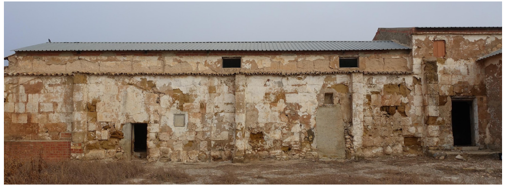
Figure 7. Southeast elevation of the main hall (Phase 3, A102, SU1001); collapse of the upper part of the walls (Phase 4, A108, SU1005); opening of the access door to the southeast house (Phase 6, A121, SU1002); destruction of the mihrāb (Phase 6, A120, SU1008); and raising of the hall (Phase 6, A114, SU1007). For stratigraphic sequence see Figure A1.
