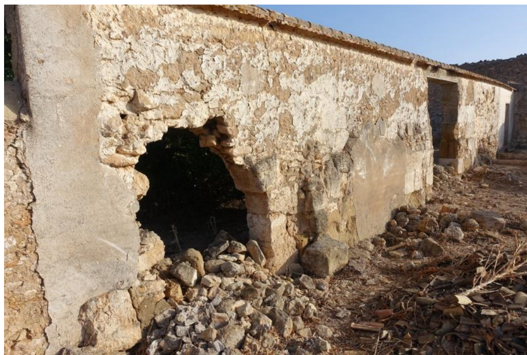
Figure 19. Northwest arcade (Phase 3, A106) seen from the south, with detail of the T-shaped pillar (SU1064) and horizontal break in the supports (Phase 4, A110, SU1057). For stratigraphic sequence see Figure A7.
