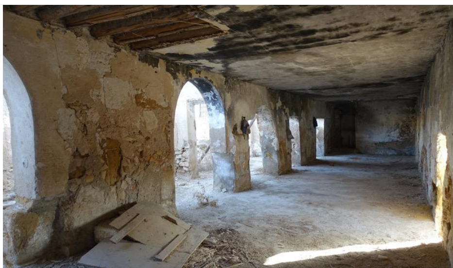
Figure 10. Interior of the southeast nave, view from the south, and arcade separating the parallel nave (Phase 3, A102, SU1077). On the right, original lintelled opening in the wall.
