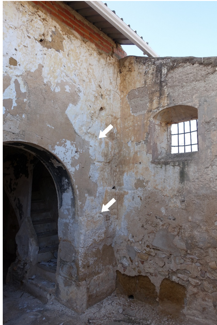
Figure 11. Junction between the interior arcade of the hall (Phase 3, A102, SU1077) and the southwest façade wall (Phase 3, A102, SU1025); remains of the carved alfiz in the corner, pointed by the arrows.
