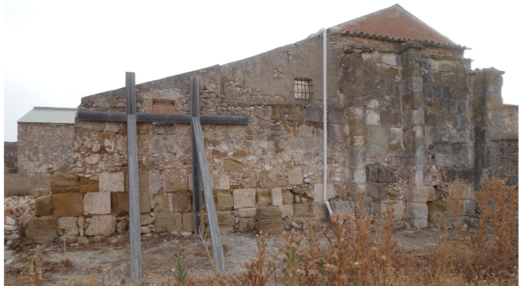
Figure 8. Southwest front of the main hall (Phase 3, A102, SU1025), ruin of the latter (Phase 4, A107, SU1037), and south house of the central courtyard (Phase 6, A117, SU1040). For stratigraphic sequence see Figure A2.
